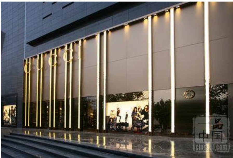
Haupteingang des neuen Gucci Shops in "The Future Mall"
